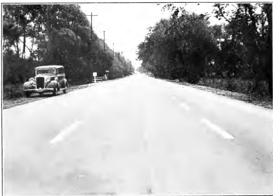
Asphalt Pavement, Highway No. 11, Showing Widened Pavement.
